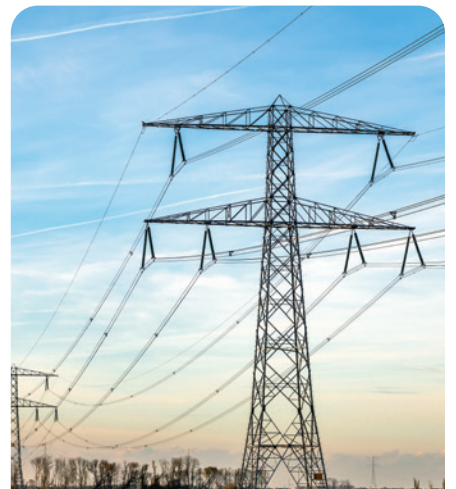
Ensuring Reliable ENERGY PRODUCTION & SUPPLY
